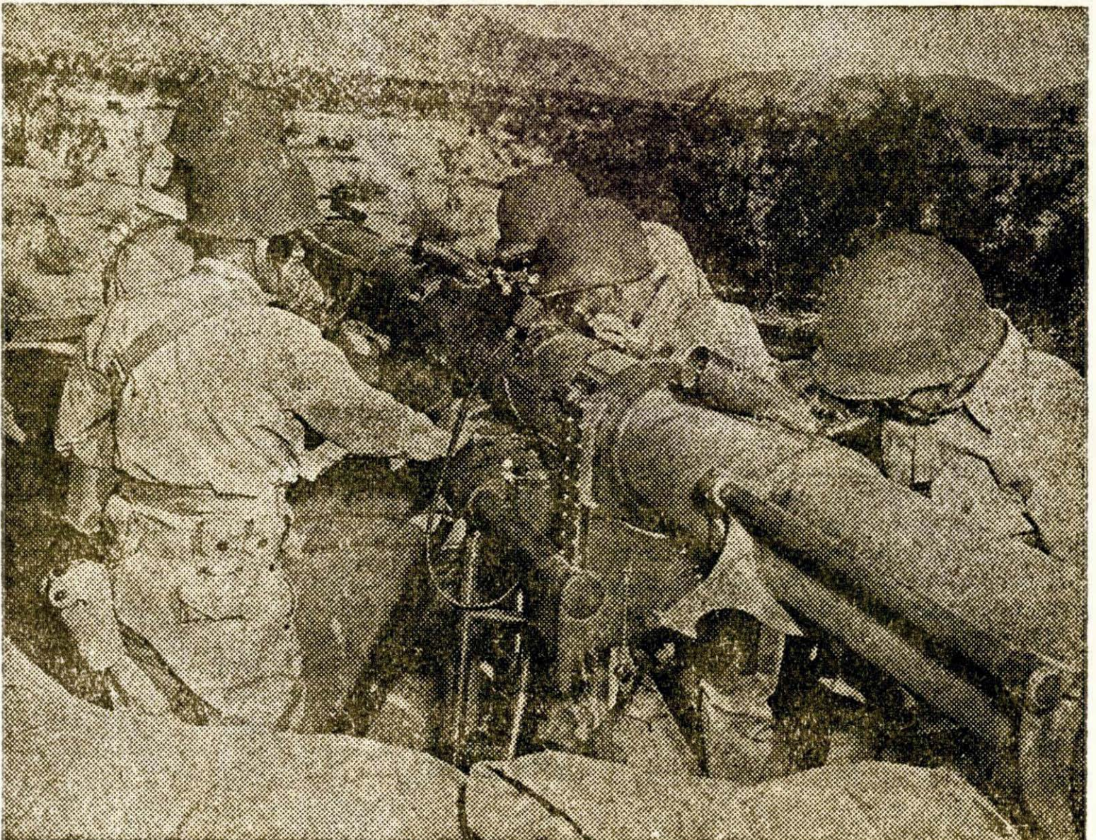
U.S. Army Signal Corps Photos Anti-aircraft range finder used to determine position of enemy planes.
